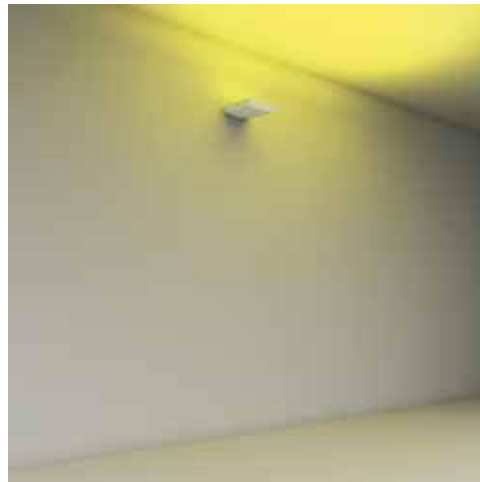
Installation on walls, ceiling washer.
